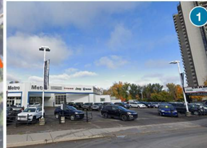
Looking north towards subject site
