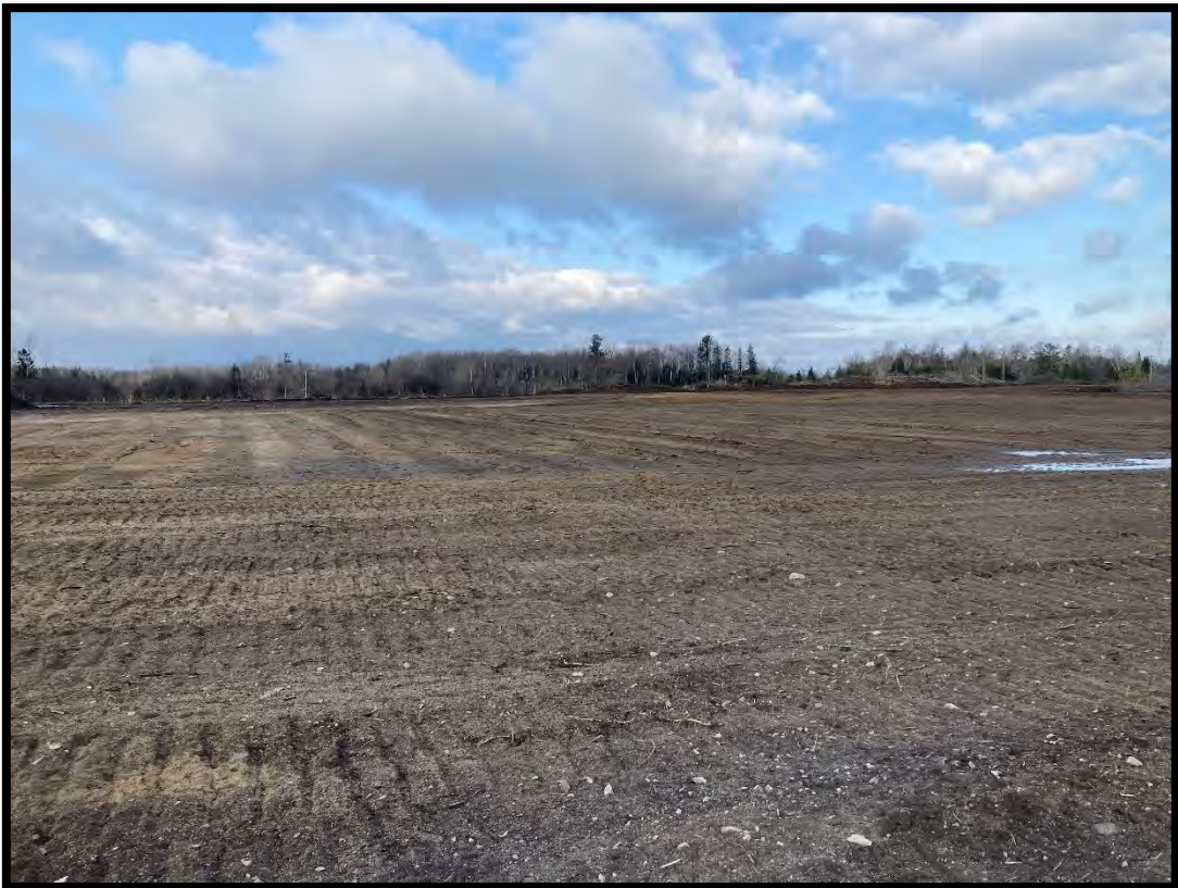
Figure 6: General view of study area, showing stripped soil and bulldozer tracks. (MH1174-D077)
