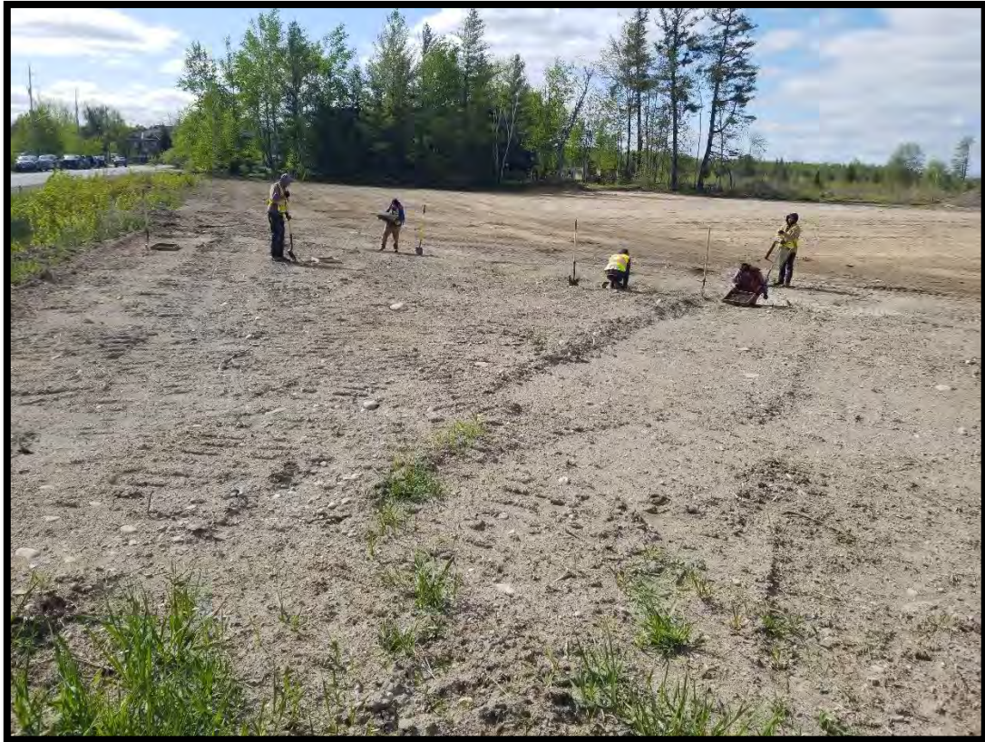
Figure 15: Test pitting in progress. (MH1174-D081)
