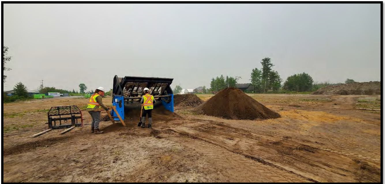
Figure 20: Mechanical sample screening in progress. (MH1174-D099)
