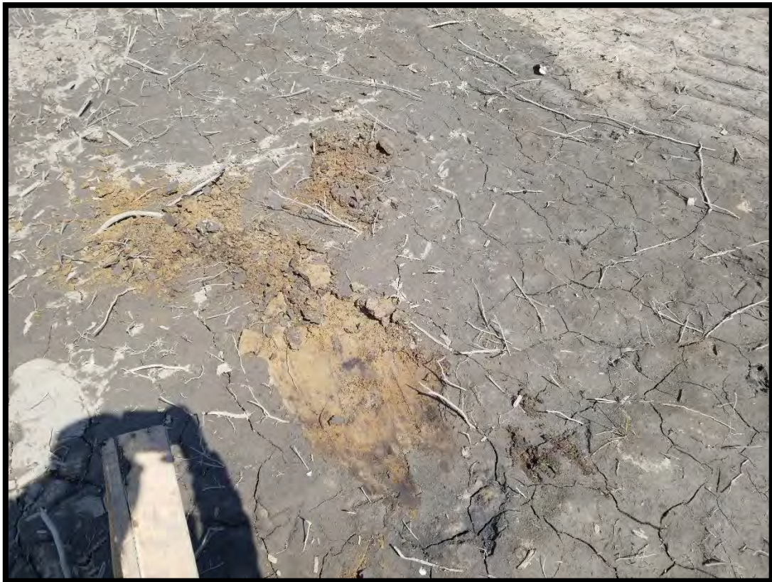
Figure 16: Example of shovel shining shallow topsoil remaining. (MH1174-D083)
