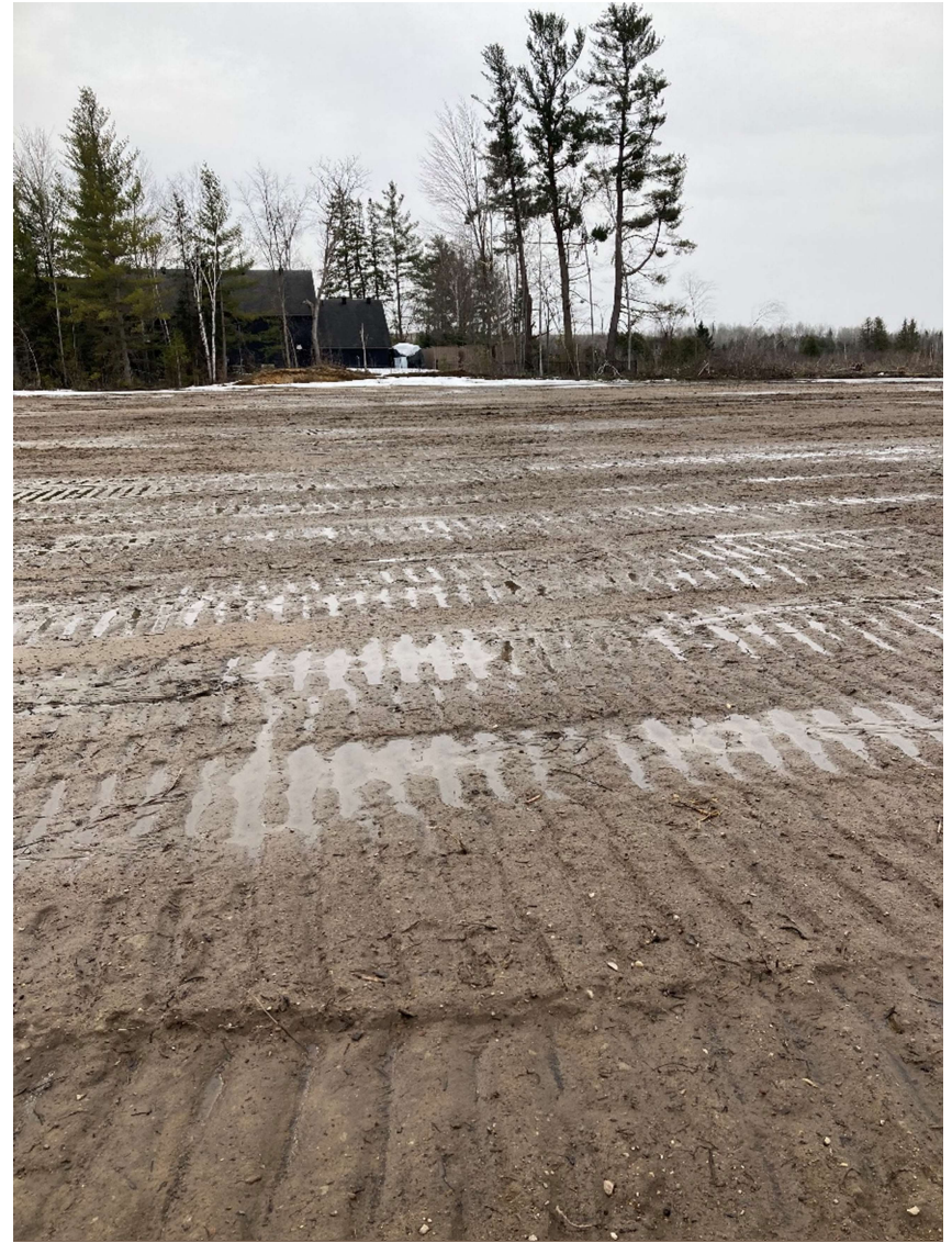
Photograph 4: Overview of 151 Wescar (looking southeast)
