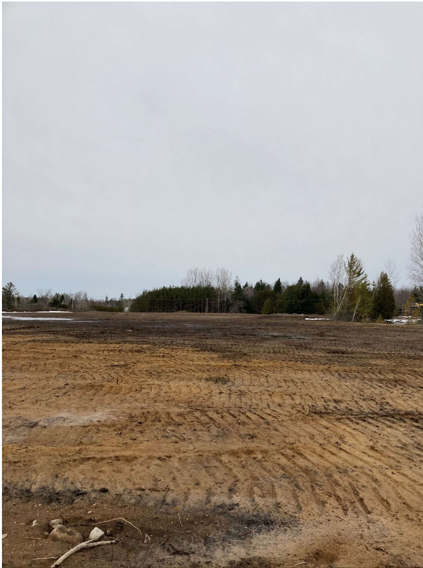
Photograph 5: Overview of 159 Wescar Lane (looking northwest)
