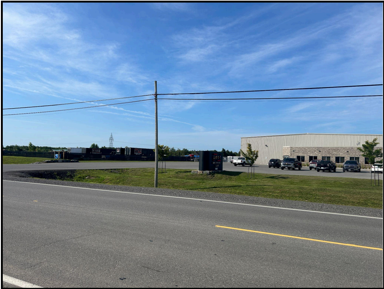
2. Front view of the existing building at 6622 Bank and the associated office space.
