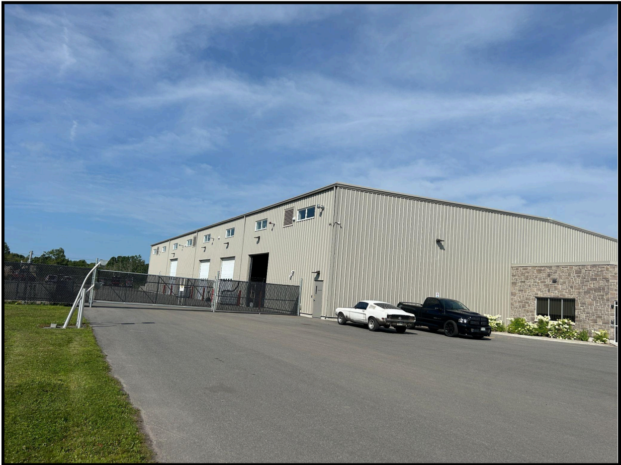
3. Internal view of the subject site looking at the existing warehouse.
