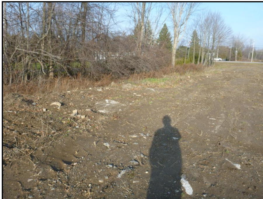
Image 14. View of stripped topsoil along the northern edge of the property prior to the addition of fill, facing northeast. (PR16-42D006)
