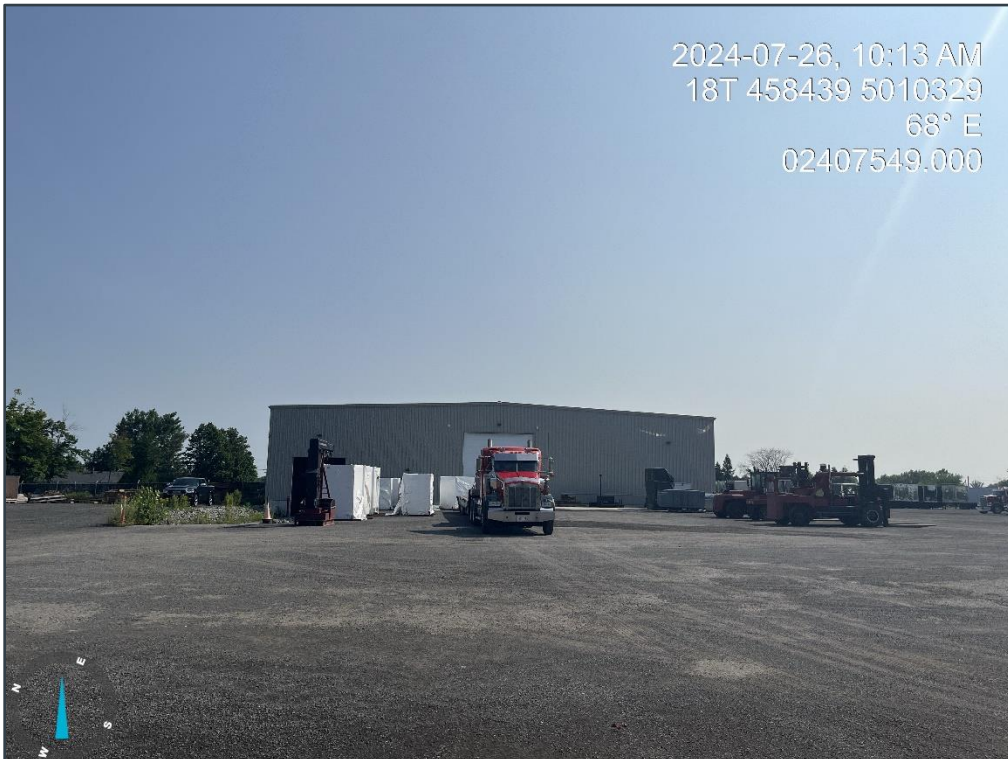
Photograph 20: Exterior West Wall of Warehouse (6622 Bank Street).
