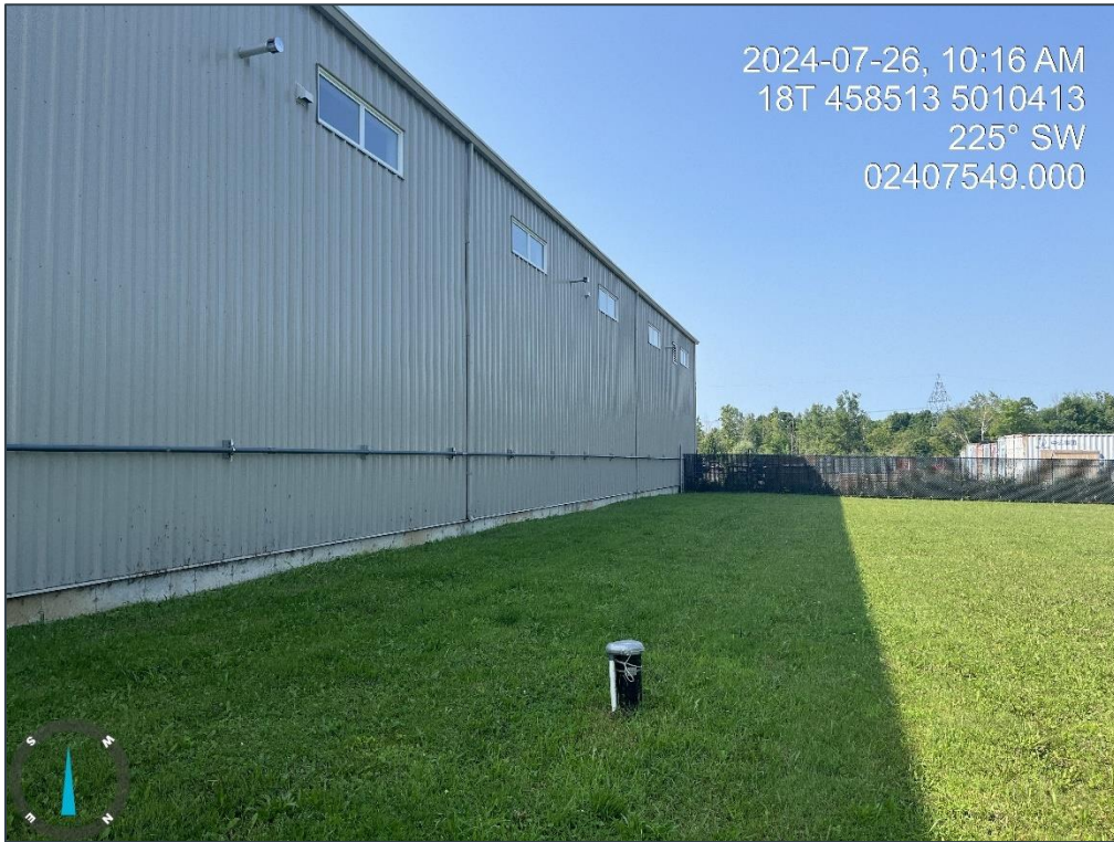
Photograph 9: Potable Water Supply Well (6622 Bank Street).
