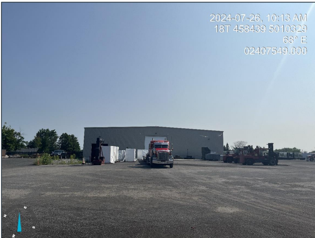
Photograph 20: Exterior West Wall of Warehouse (6622 Bank Street).
