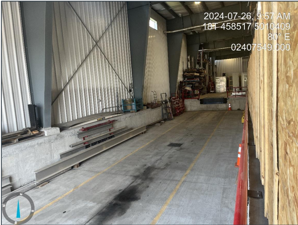
Photograph 5: Interior Warehouse Loading Dock Area (6622 Bank Street).
