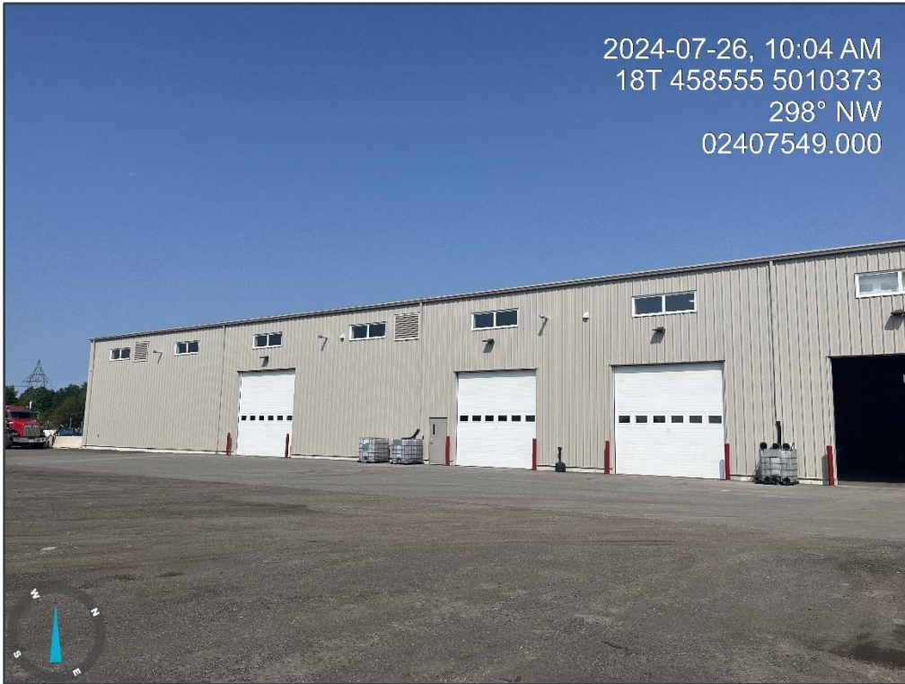
Photograph 19: Exterior South Wall of Warehouse (6622 Bank Street).
