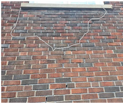
4. Staining of the brick under windows indicates long term water running down the face with cracking from the upper to the lower window.
