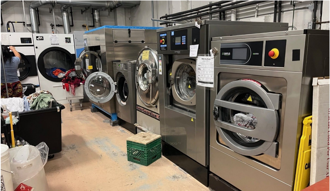
Figure 7 Photo of laundry machines in existing cleaning location on Sheffield Road in Ottawa
