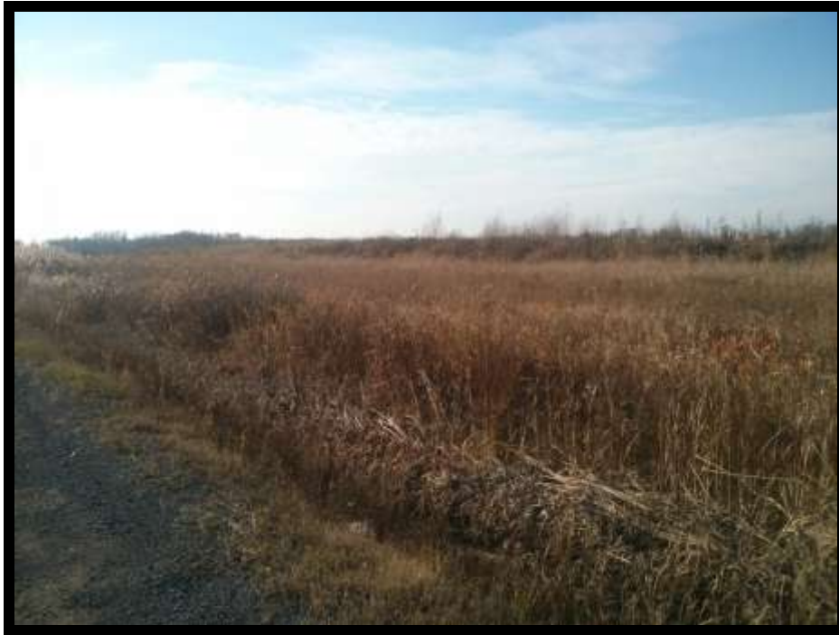
Photograph 1: View of the raised fill layer that encroaches on the subject property, facing north.
