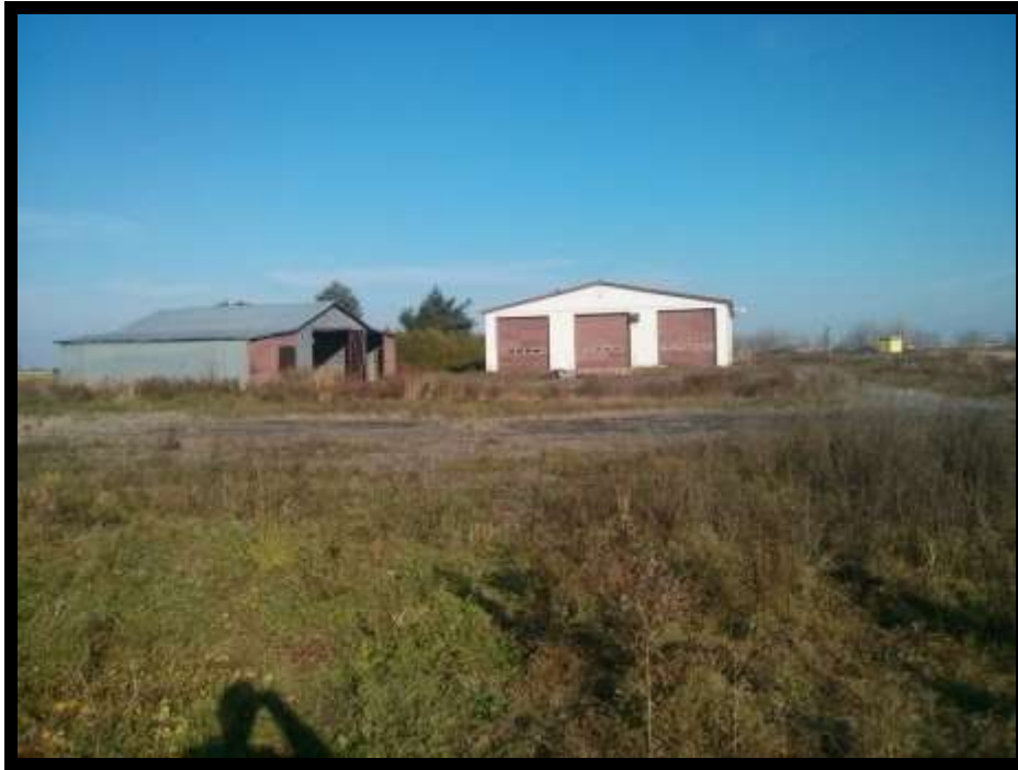
Photograph 3: View of the former welding shop, facing east.
