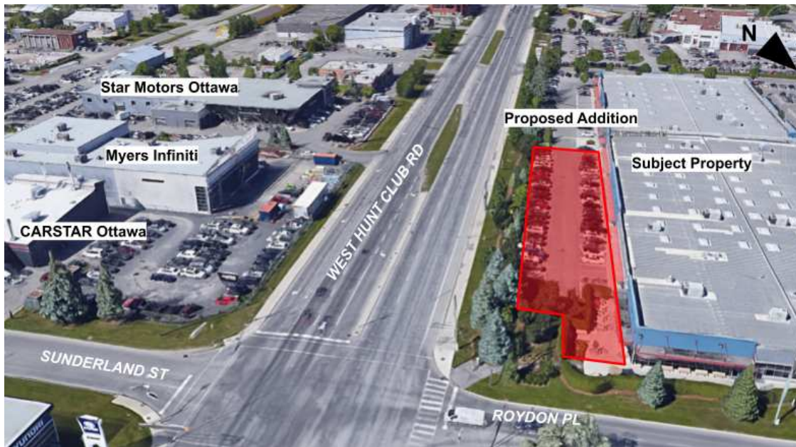
Existing streetscape of West Hunt Club Road looking southwest.
