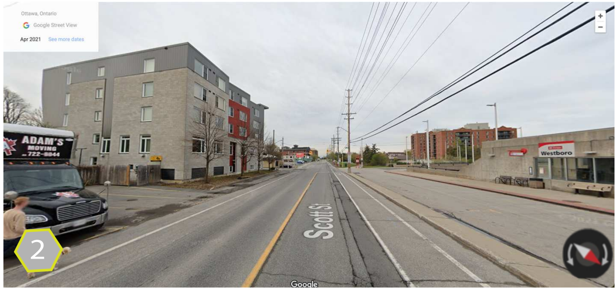
Figure 18: Photo 2: View looking southwest along Scott Street (Source: Google Maps)
