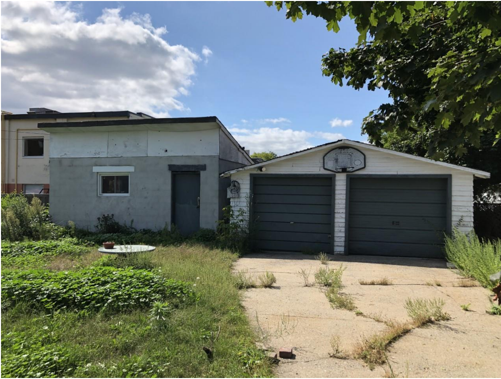
Photograph 3: View of the car garage and storage shed, facing west.
