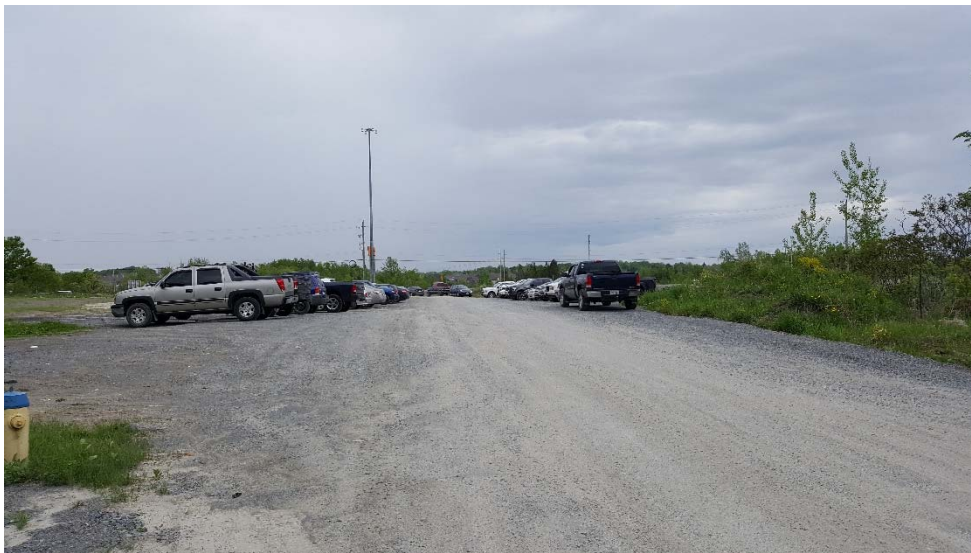
Photo 4 - View of the north portion of the Site facing east. View depicts temporary granular gravel fill as construction parking area.
