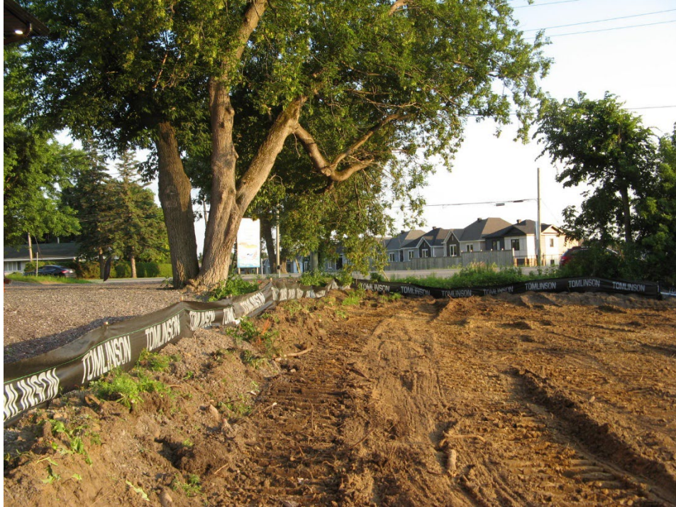
Photo 3 – Silt fencing and initial regrading adjacent to Tree ‘A’. View looking south to Navan Road
