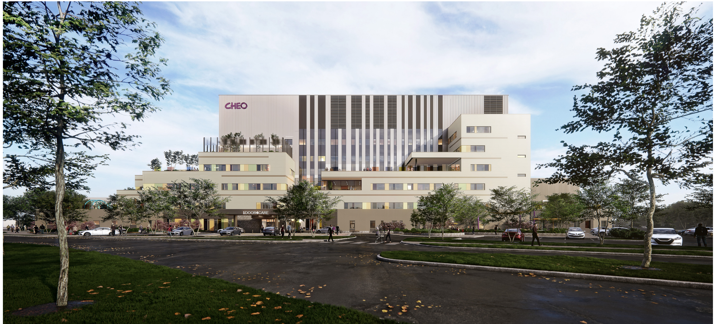
Ground view of 1Door4Care south elevation – approaching from Smyth Road
