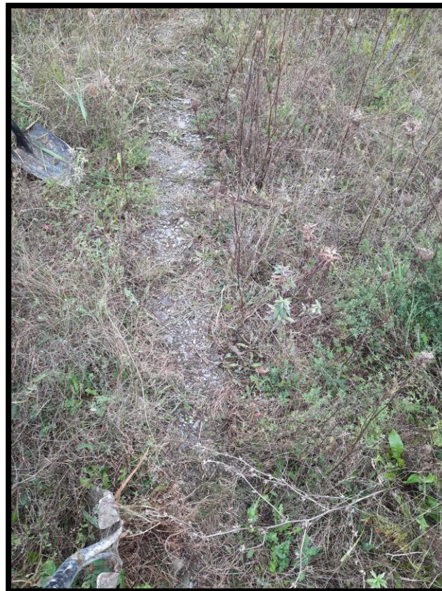
Figure 10: Gravel on surface, western boundary (D031).
