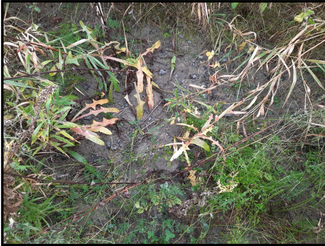
Figure 9: Gravel on surface, western boundary (D030).
