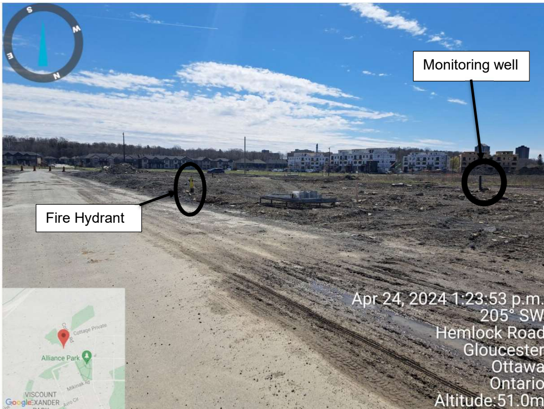
Standing at northeast side of Oshedinaa St. and looking towards southwest of Block 6 and Block 5 : No indications of existing slope greater or equal to 2 m in height or any settlement. Presence of service lines, monitoring wells, etc.
