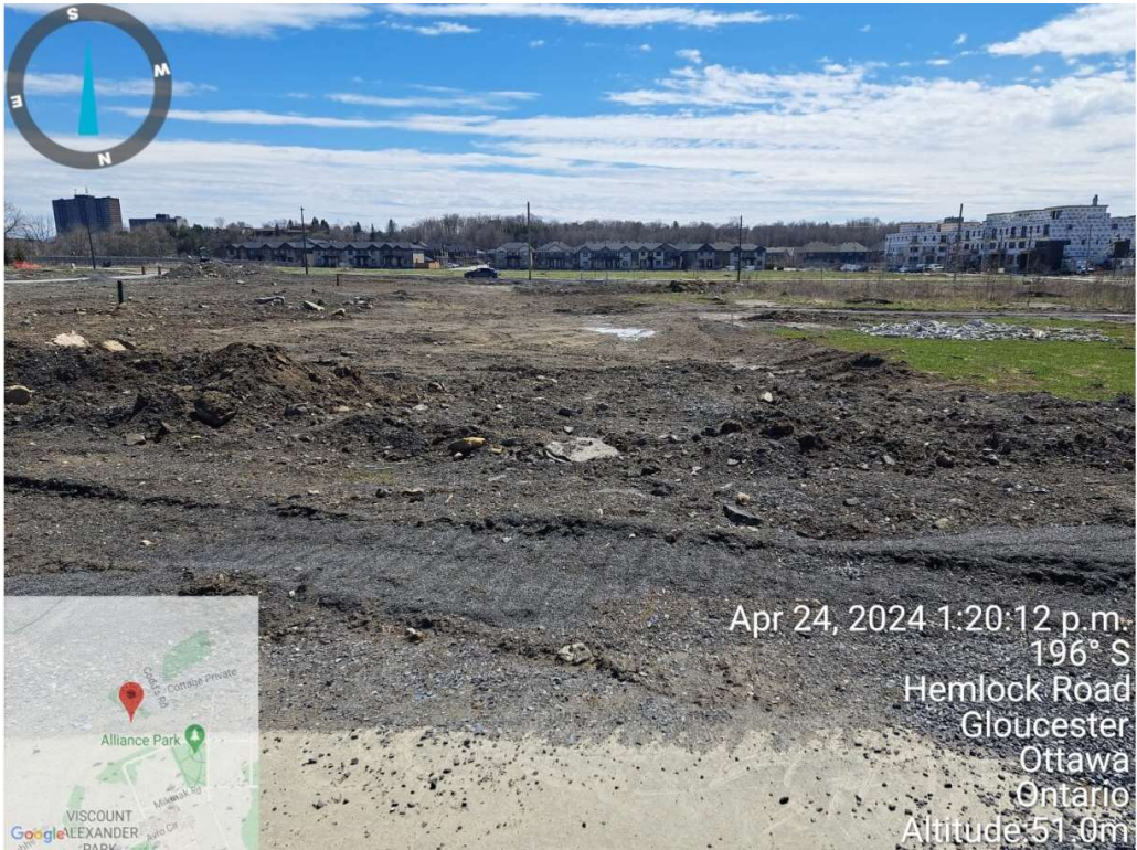
Standing at northside of Street No.1 and looking towards south of Block 5 : No indications of existing slope greater or equal to 2 m in height or any settlement.
