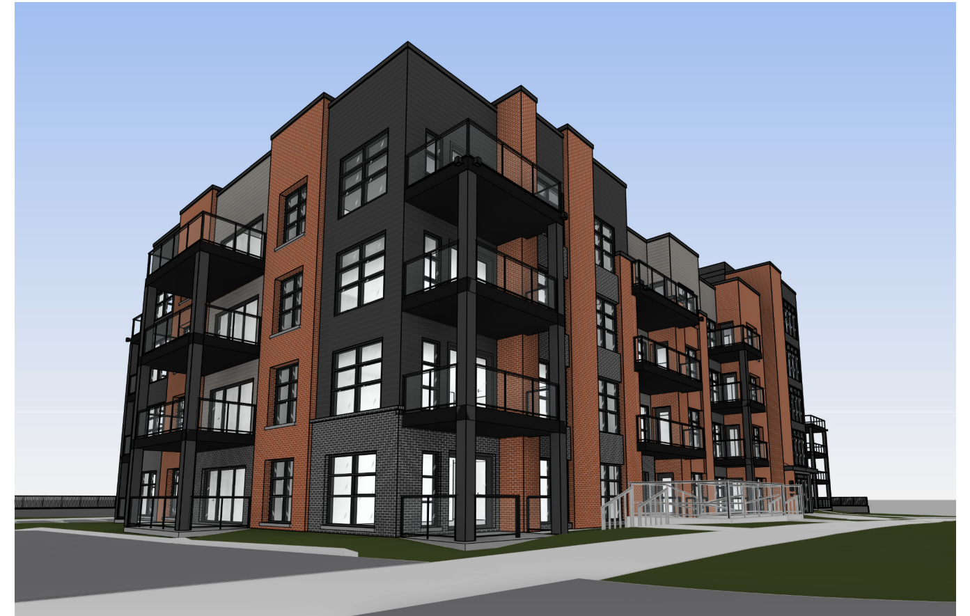
Figure 7.5 – Looking northwest towards Building C along Oshedinaa Street (September 2024).
