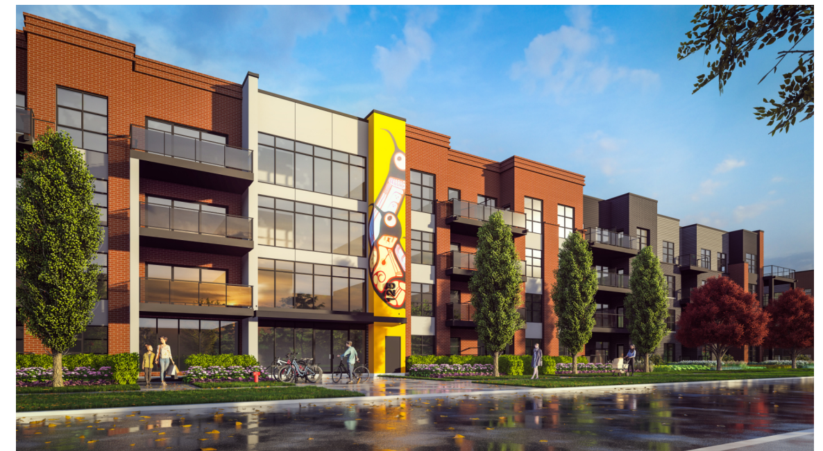
Figure 13.1 – Looking northwest towards the main entrance of Building B (September 2024).
