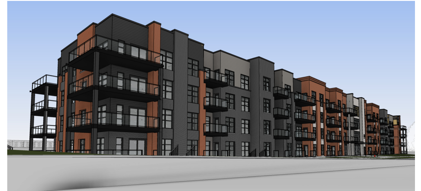
Figure 7.1 – Looking northwest towards Building B along Oshedinaa Street (September 2024).
