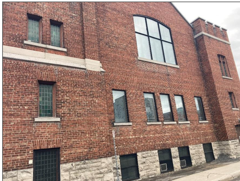
Photo 4 – Site Building (southwest elevation).
