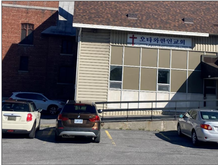
Photo 3 – Site Building (southeast elevation).
