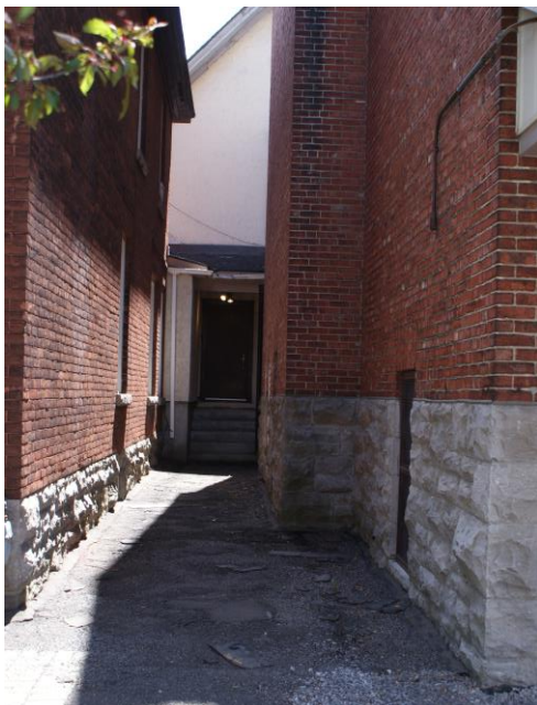
Figure 12: View of the coursed limestone foundations of the 1910 Church (right) and the 1902 Parsonage (left). Note the difference in the stone module (size and finish) between the front and side elevations of the church. The stone from the demolished foundation walls will be used to accommodate changes to the grade level windows in the Bell and Arlington facades. The limestone foundation walls of the Parsonage should be salvaged for potential landscape use. Source: Commonwealth 2024
