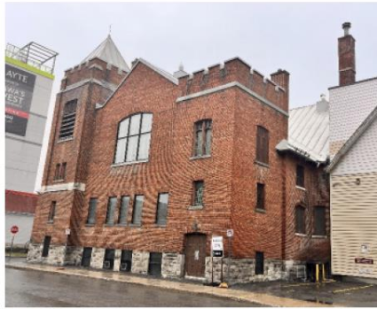
Figure #2: Heritage Façade along Bell Street [JCAL 2024]
