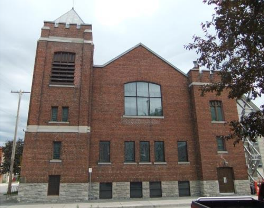
Figure 8: View of the west Bell Street façade of the 1910 United Church. The six (6) art/stained-glass windows in the west façade are intact and have been protected with recently installed double glazing units. Source: Ontario Heritage Trust.
