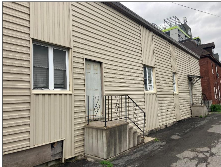
Photo 2 – Site Building (northeast elevation).
