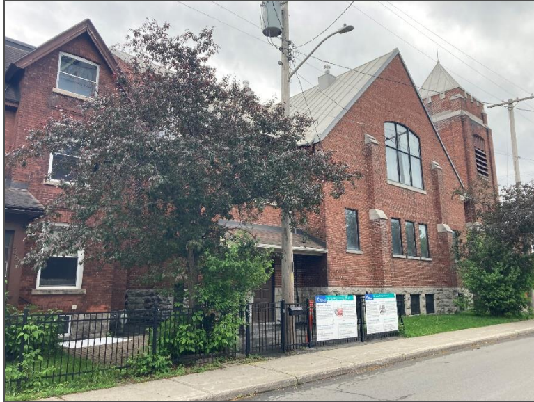
Photo 1 – Site Building (northwest elevation).
