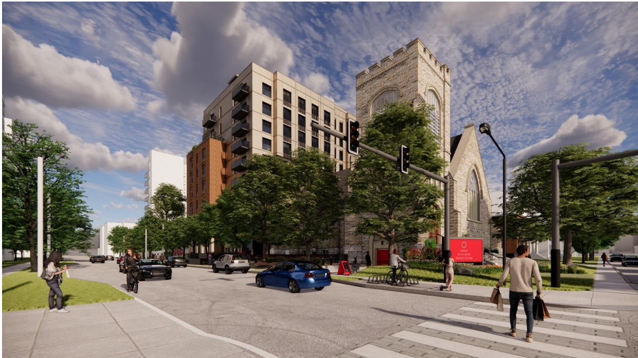
Figure 16: The vertical emphasis and pivot point of the church's tower is continued on the corner of Laurier and Blackburn Avenues with a brick tower element. This new corner acts as a transition from the institutional language of the church to the residential condition and language of the surrounding neighbourhood. The material transition to brick also acts as a subservient nod to the stone of the church.
