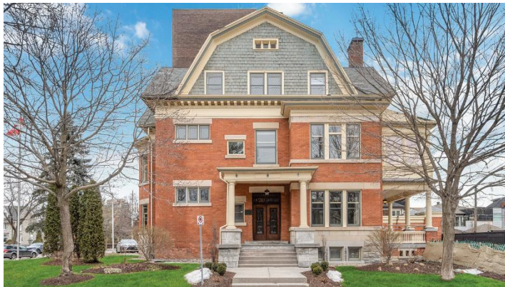
Figure 12: Street view of 5 Blackburn Avenue. Source: Google Earth May 2021
