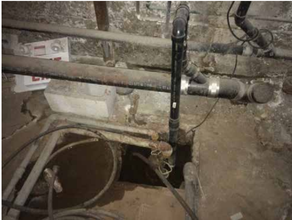
Photograph 15. View of a sump pit, located in the mechanical room of the church
