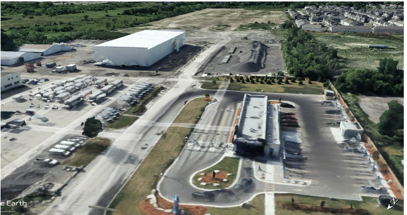
View of Neighbouring Car Wash from Street Entrance
