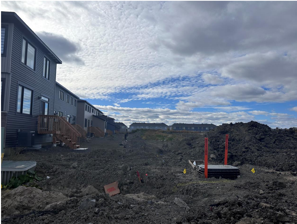
Figure 2 South-east corner of the site looking west
