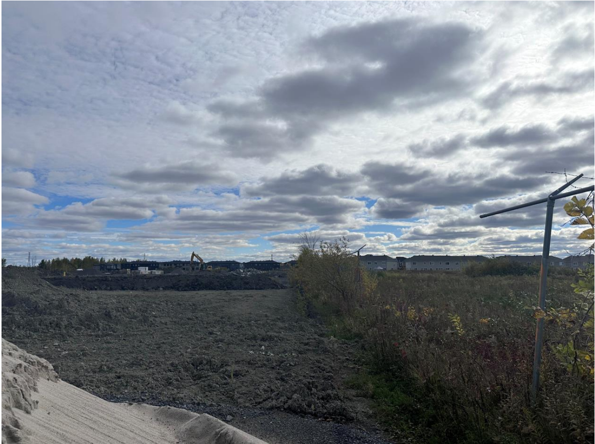
Figure 1 North-west corner of the site looking south
