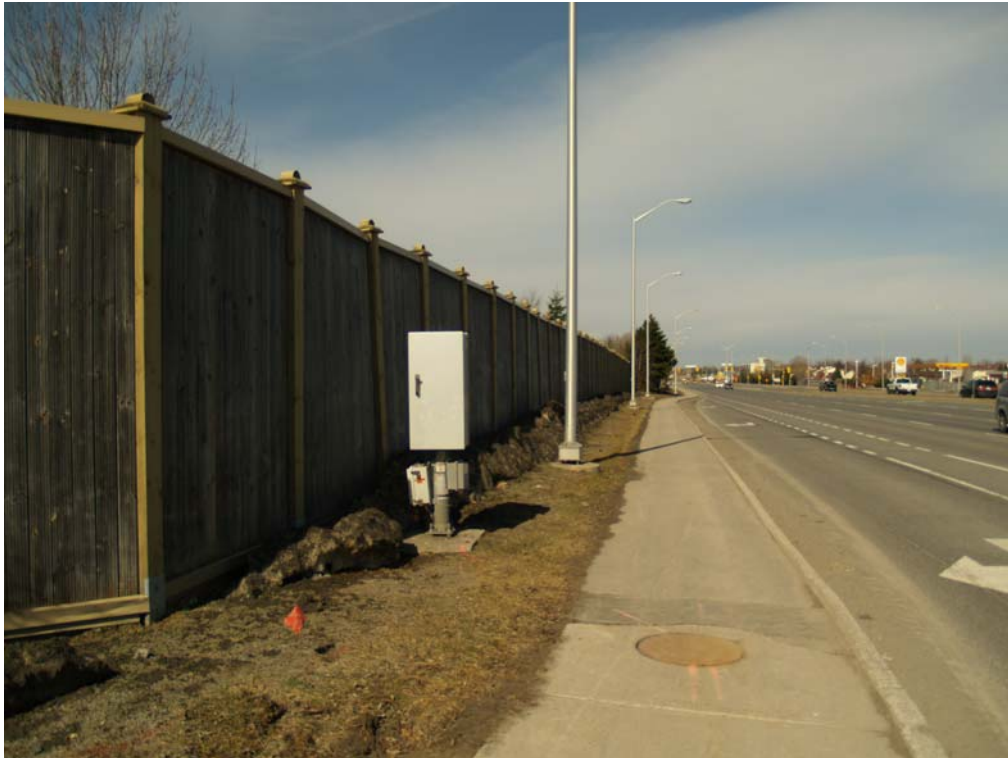
PHOTOGRAPH 3: EXISTING CONDITIONS – TERRY FOX AT MARCH (RECEPTOR 8)
