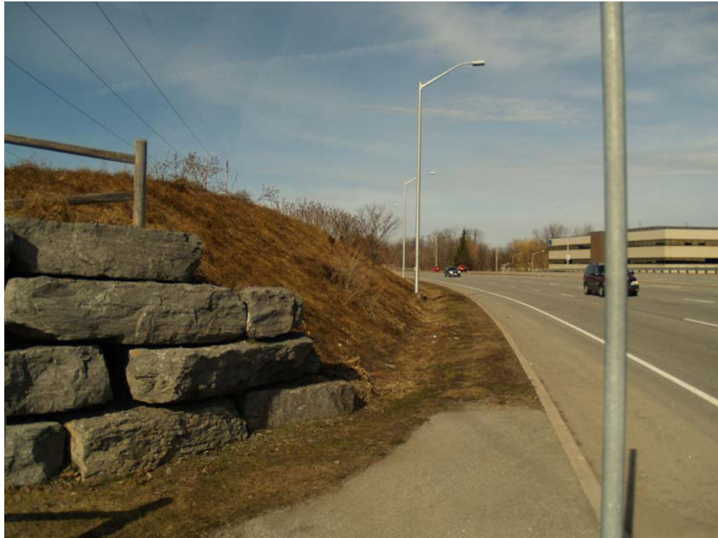
PHOTOGRAPH 2: EXISTING EARTH BERM ALONG MARCH ROAD
