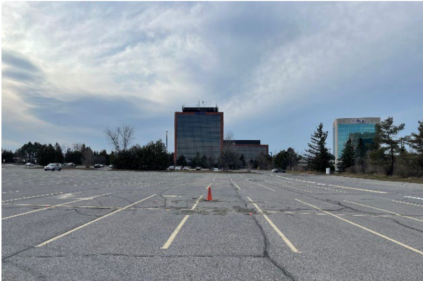
2. Nokia campus parking lot looking Northwest
