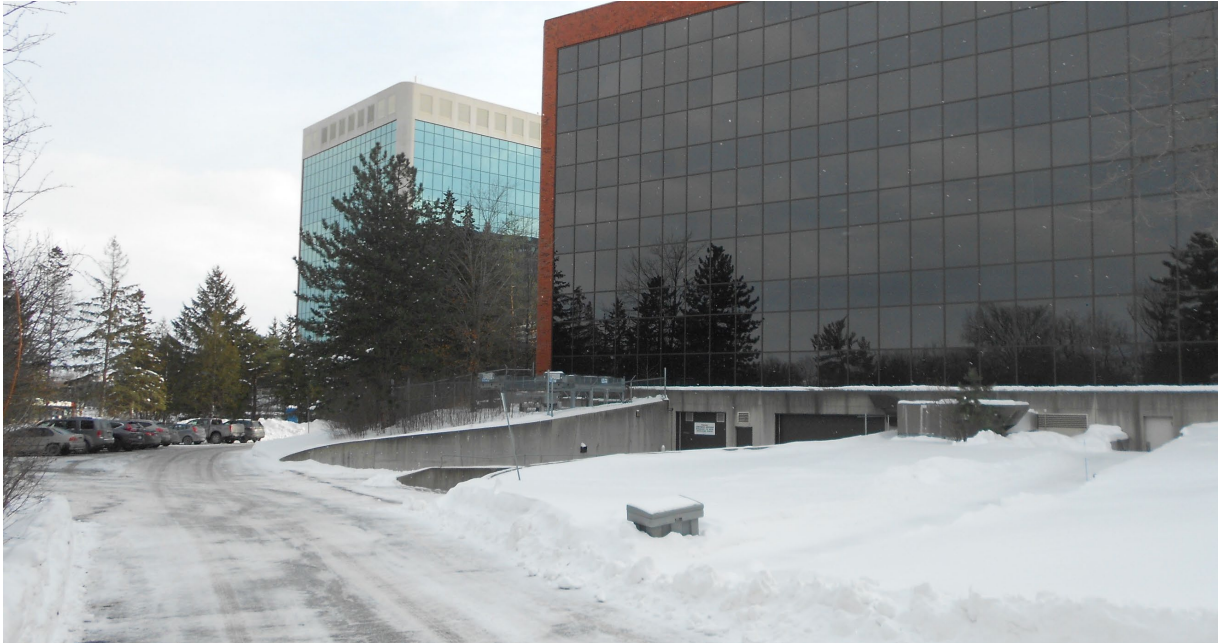
Photo 5 View of Site Building (Tower 2) with ramp to below ground parking, facing east.
