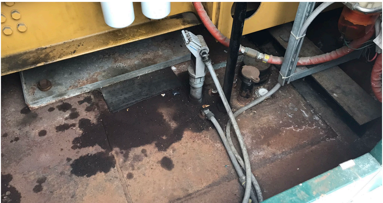
Photo 26 Evidence of drips/staining below generator (on top of decommissioned flat tank) in outbuilding located in the northeast portion of the Site.
