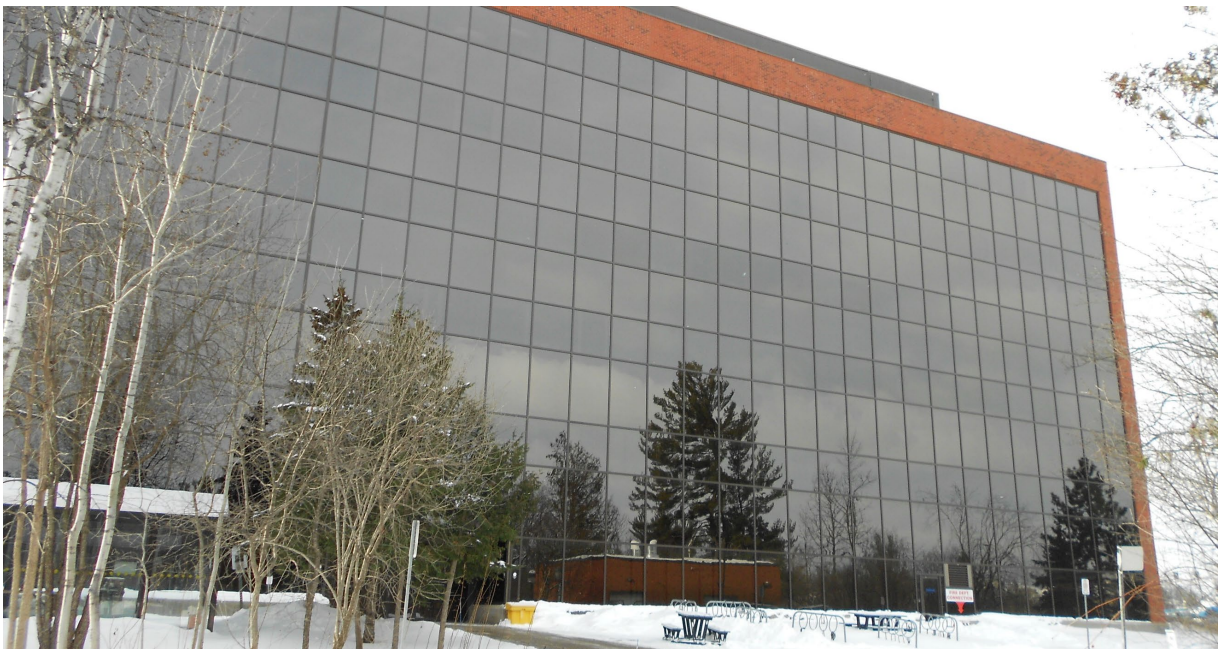
Photo 4 View of Site Building (Tower 1), facing west.
