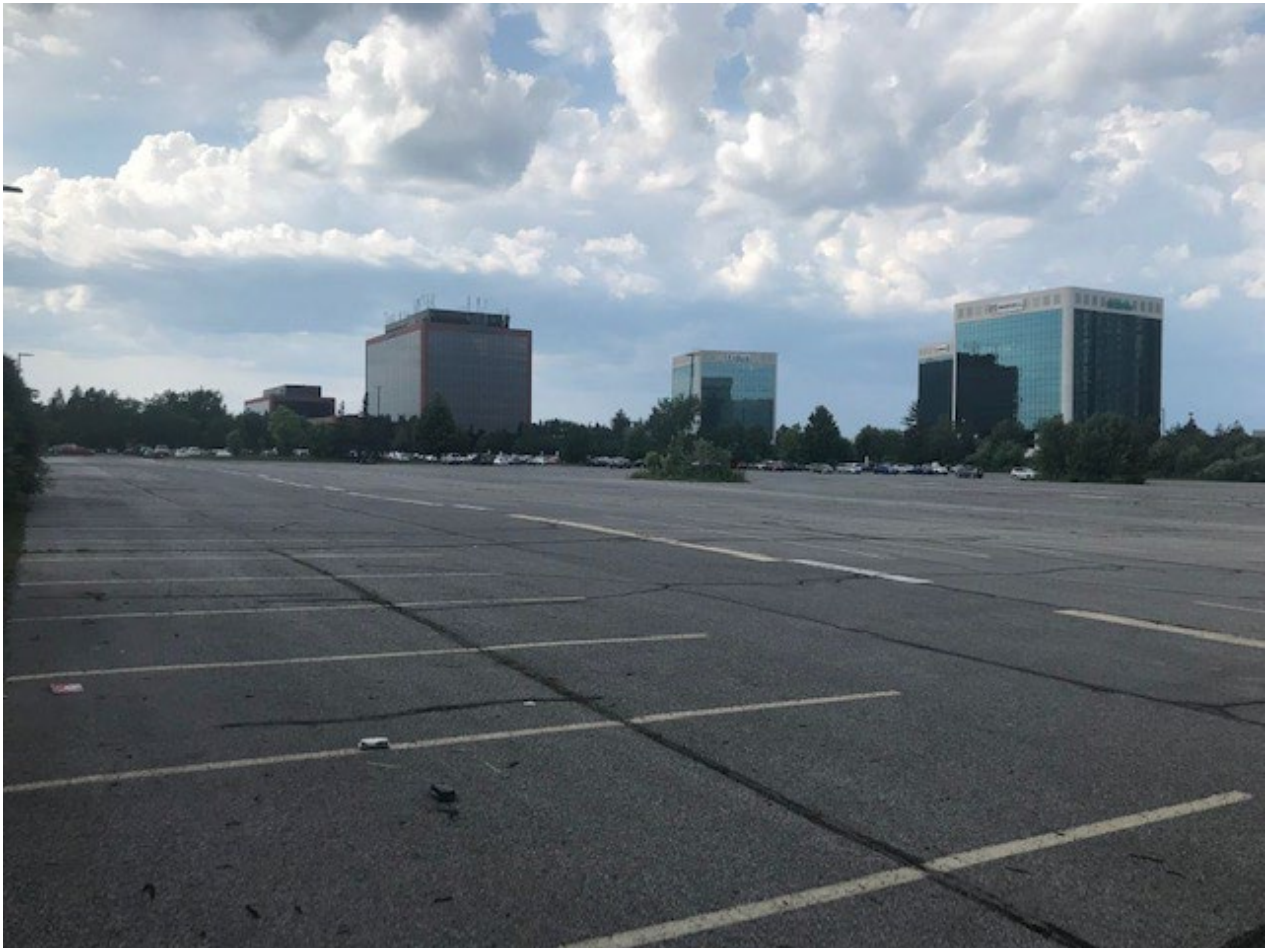
Photo 1 View of Site (Parking Lot), facing North. Adjacent Nokia office towers (left) and adjacent office towers (right; beyond Legget Drive) observed.
