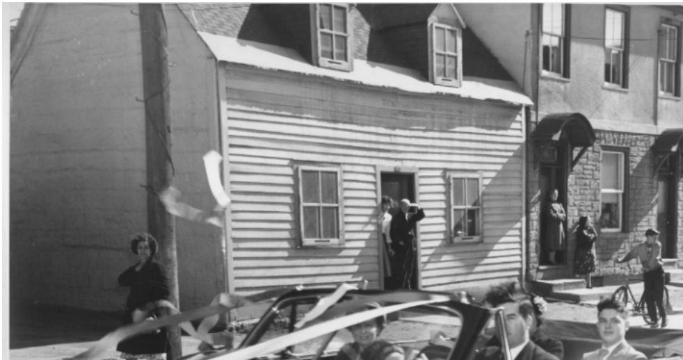
Figure 3: The house at 168 Murray appears in the background of the c.1949 parade. The house is a 1.5 storey side gable with two dormers facing the street, a centre front door with no canopy, horizontal siding on the front and squared timber chinked and whitewashed on the gabled side elevation. Source: Marc Aubin Collection.
