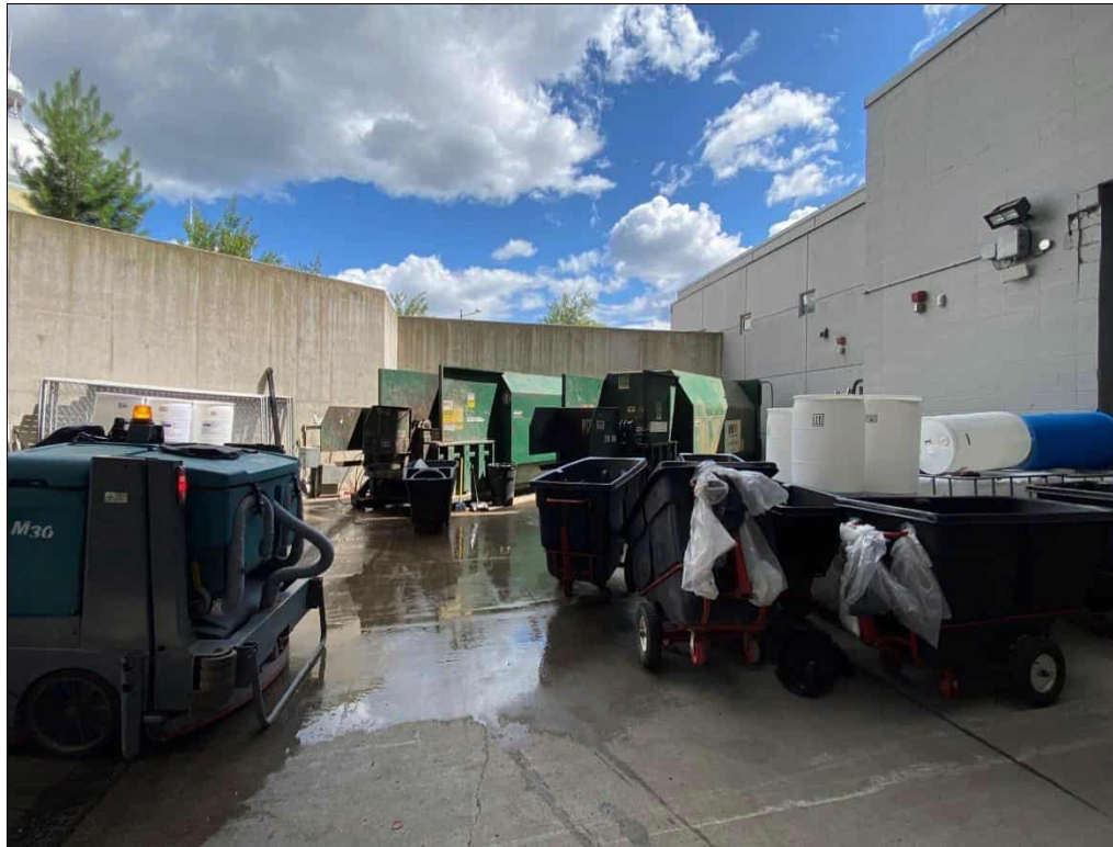
Photo 39: TD Place Stadium: Hydraulically operated garbage and cardboard compactors located at the bottom of the ramp to the loading dock area. Date: 08/01/23 Direction: Southeast
