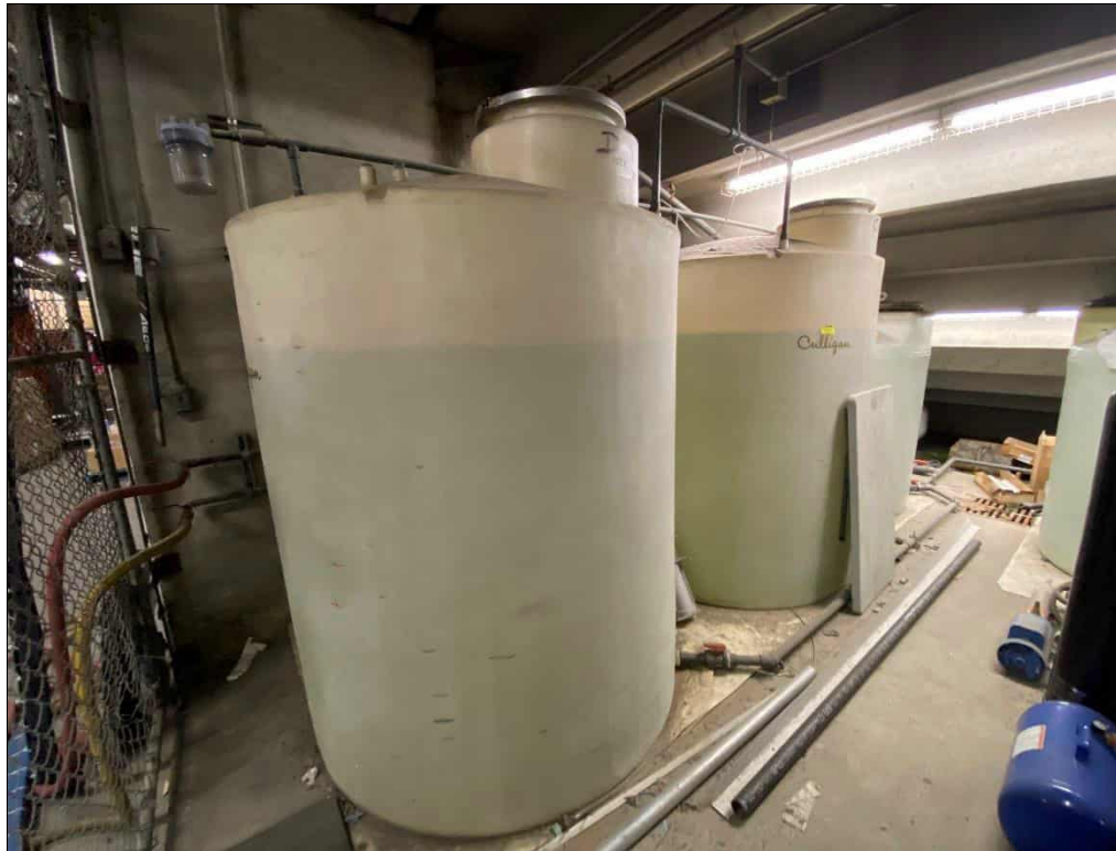
Photo 19: TD Place Stadium Service Level: Reverse osmosis water storage tanks for ice making. Date: 08/01/23 Direction: N/A
