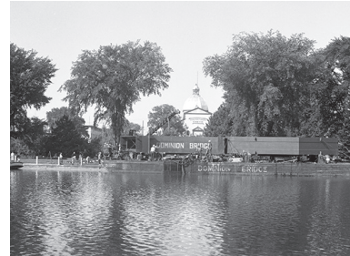
1966 Unloading steel box girders for the Frank Clair Stadium and Civic Centre from a boat on the Rideau Canal (City of Ottawa Archives).
