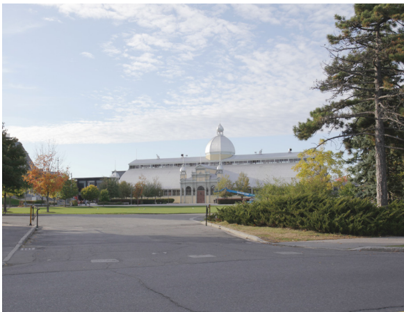
View H1.2 existing condition.
