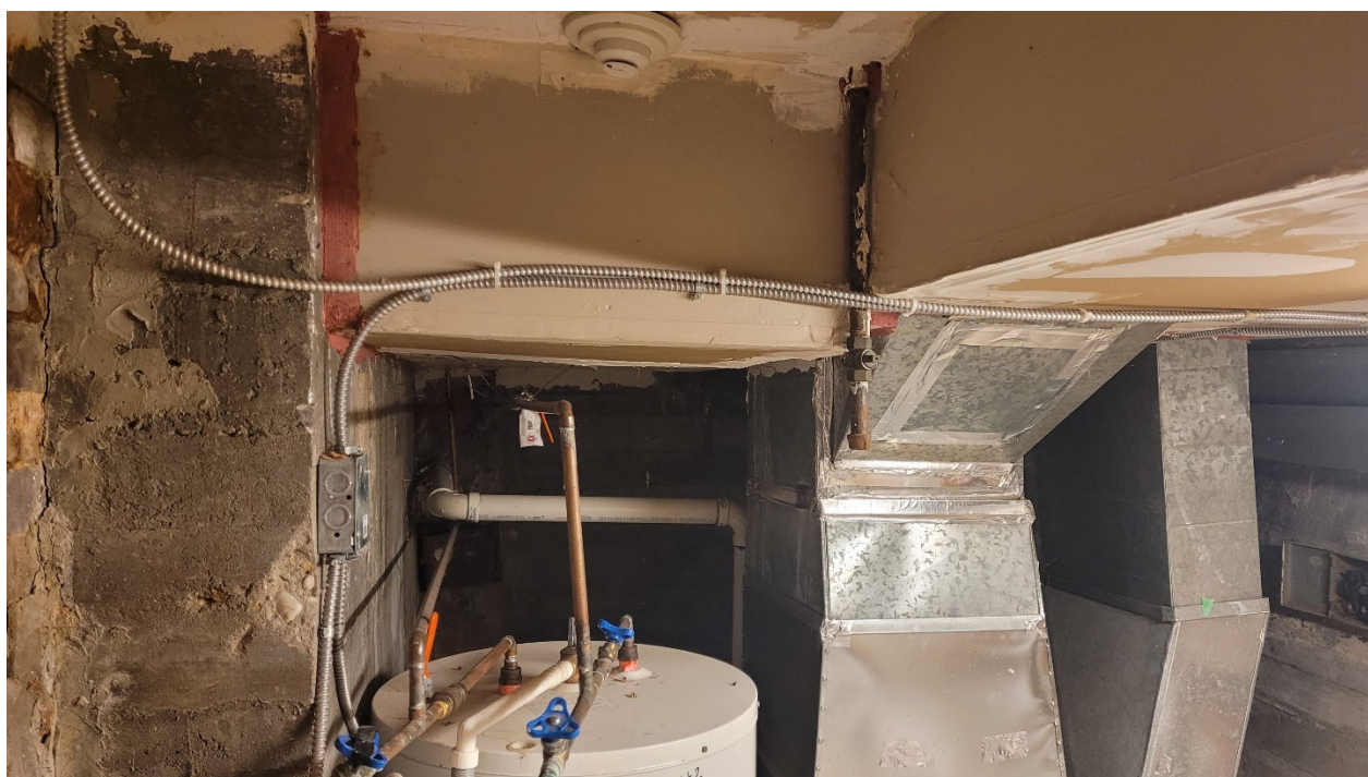
Photograph 6: View of the natural gas fired equipment, ceilings and foundation walls in one of the buildings' mechanical rooms. Note that recent drywalling around the mechanical room ceilings prevented observation of potential former heating oil supply lines.
