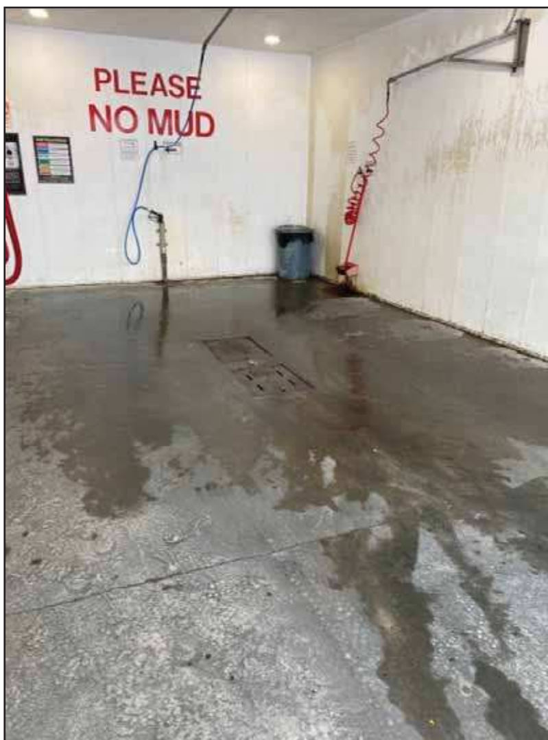
Photograph 9: Interior view of a car wash bay.
