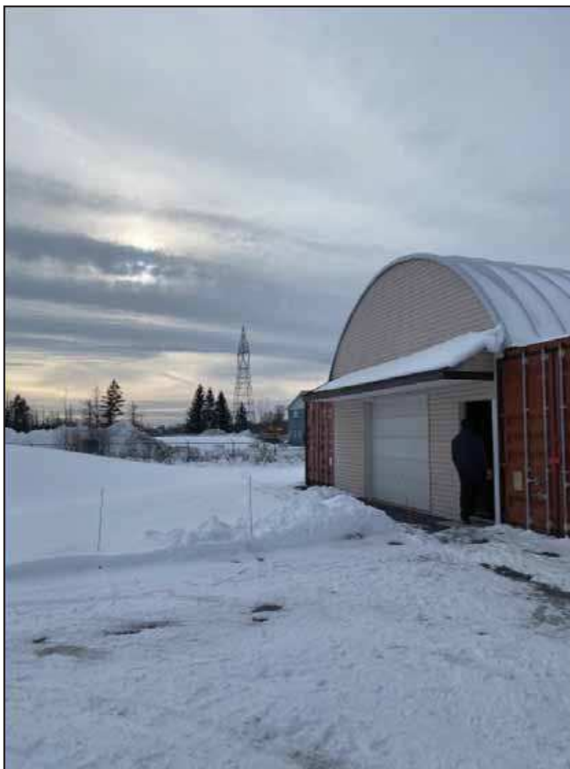
Photograph 6: View of the recently build storage building.
