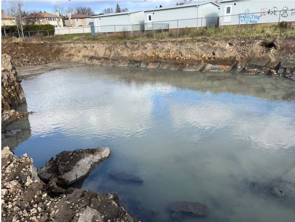
Photo 3: Significant water on subgrade in area of building A3 which was backfilled with clay and boulder fill prior to approval (November 19, 2021)
