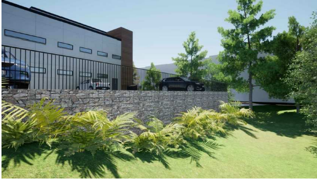
Figure 9. View of parking lot gabion wall.
