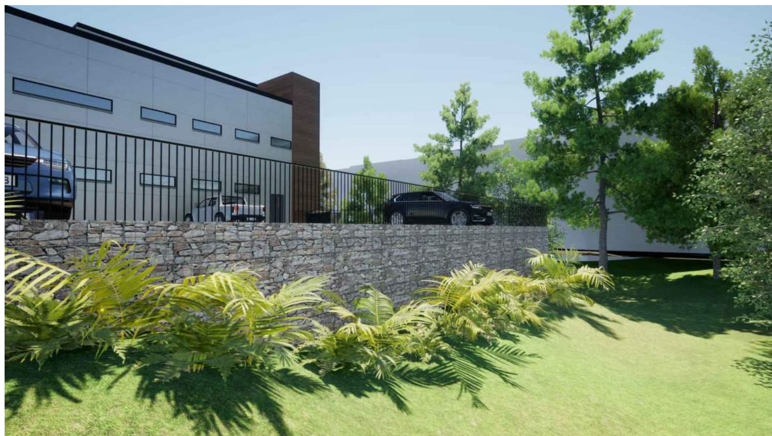
9 VIEW OF PARKING LOT GABION WALL
