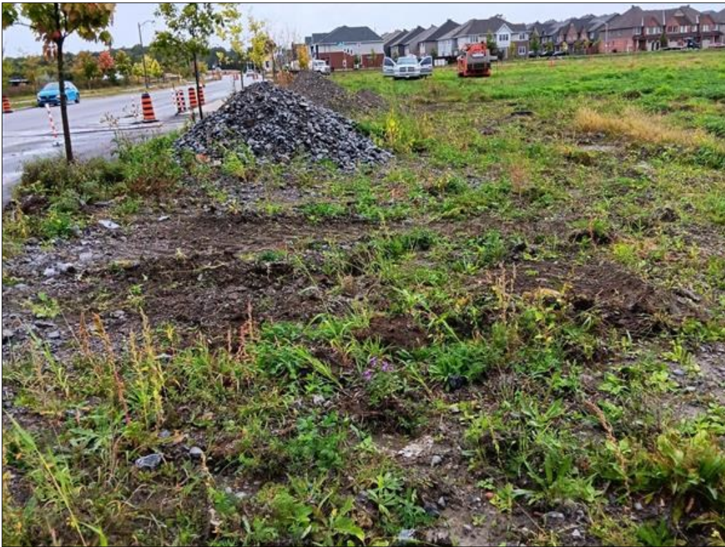
PHOTO 3 - Two stockpiles of fill material located at edge of property, adjacent to Kelly Farm Drive.
