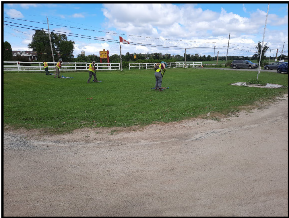
Figure 8: Test pitting in progress, (MH1289-D031).
