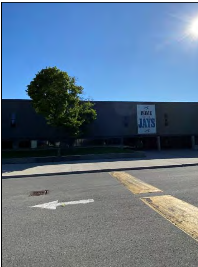
Photograph 2: Looking east-north-east at the front entrance to the subject building from the parking lot.
