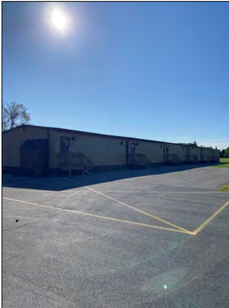
Photograph 9: View of portable classroom units on the exterior south side of the subject building.
