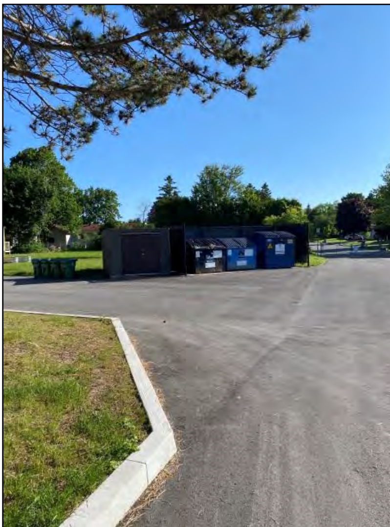
Photograph 8: View of dumpsters and a storage shed on the exterior east corner of the subject building. Paddock Way is in view on the right side of the photo.
