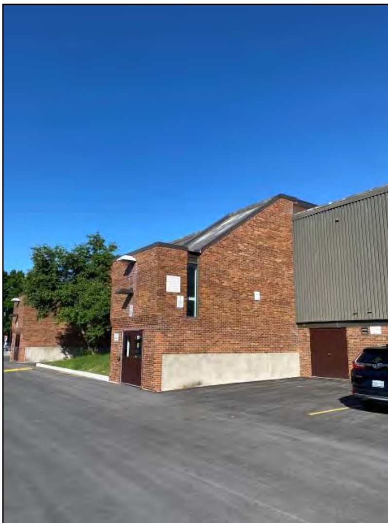
Photograph 6: View of the south building elevation (location of the proposed addition).
