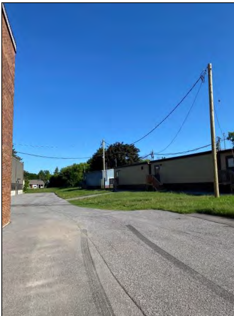
Photograph 5: View of portable classroom units on the east side of the subject building.
