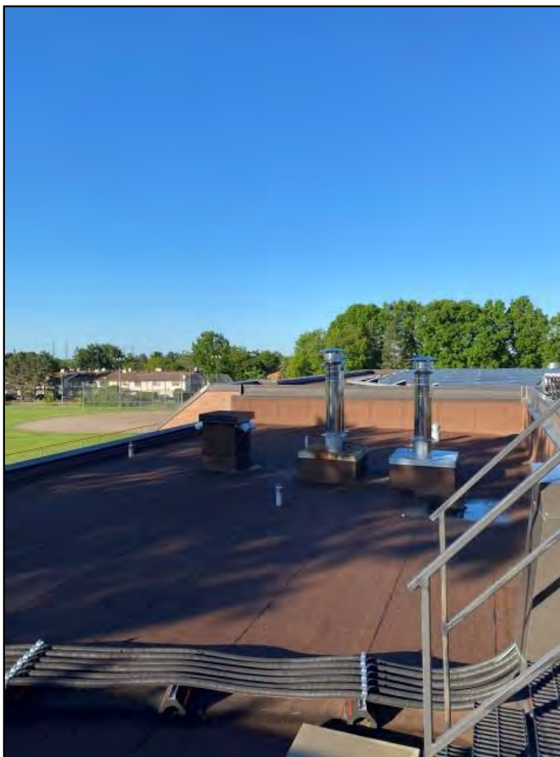
Photograph 21: View of a chimney stacks above the boiler room.
