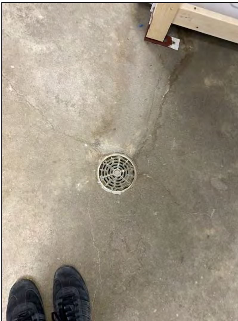
Photograph 24: View of a floor drain in custodial room 142.
