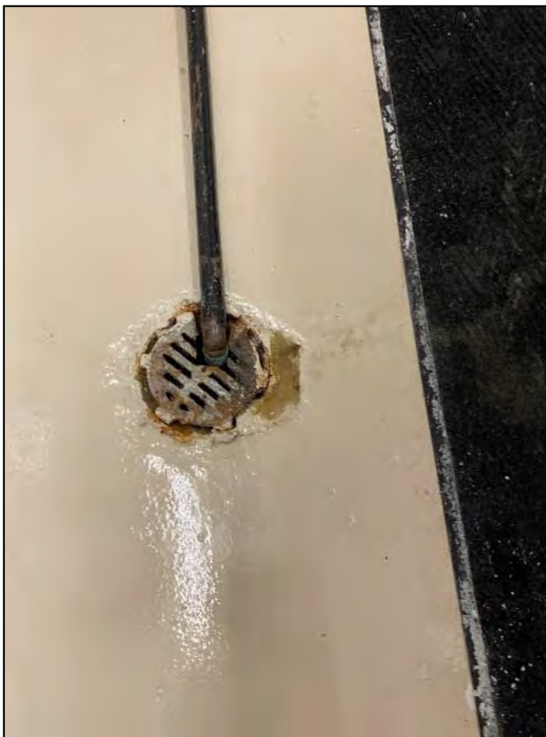
Photograph 27: View of a floor drain in room 140f.
