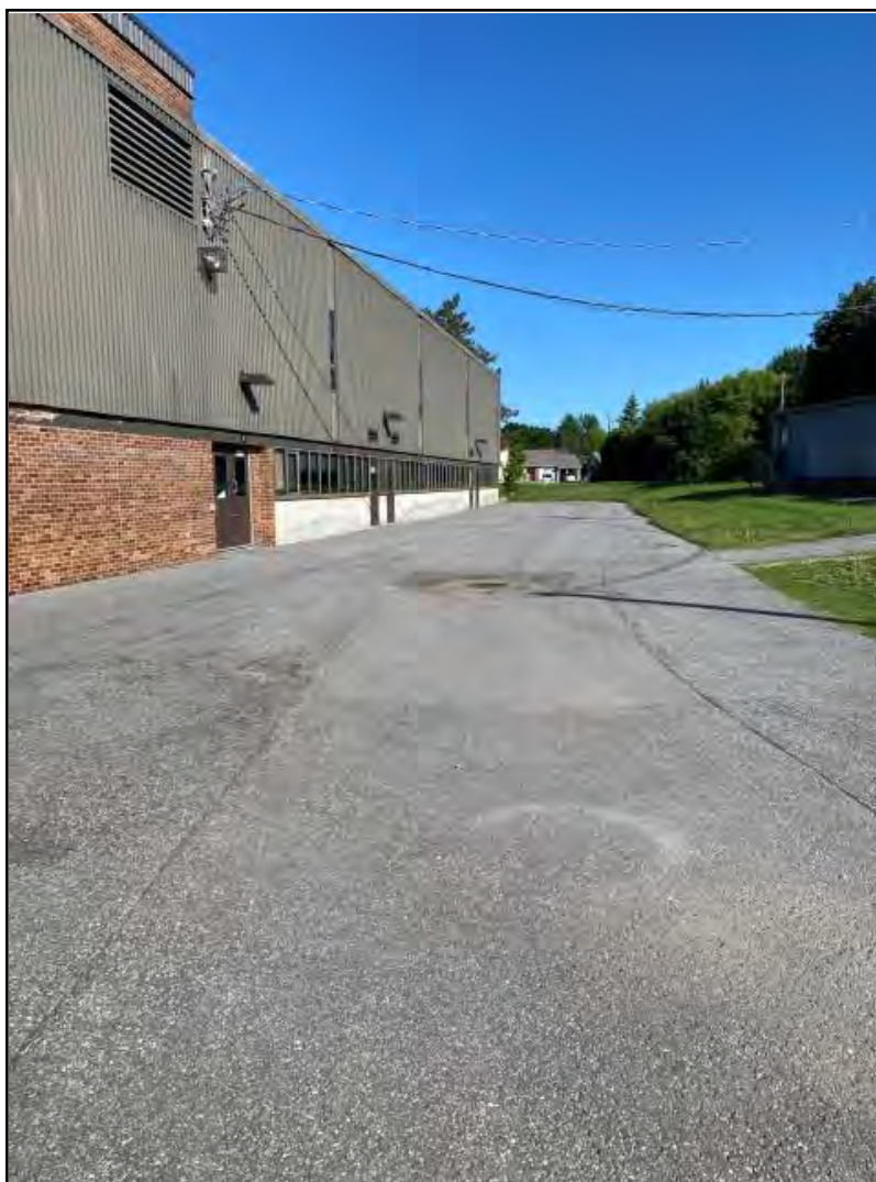
Photograph 4: View of the east building elevation. Overhead hydro and communication lines and a stormwater catch basin are in view.
