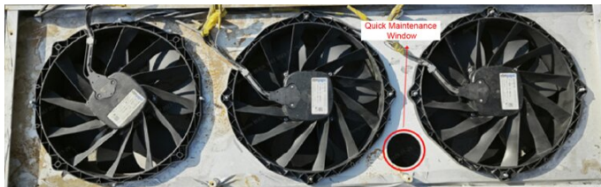
figure 5-36 Schematic Diagram of Quick Maintenance Window
