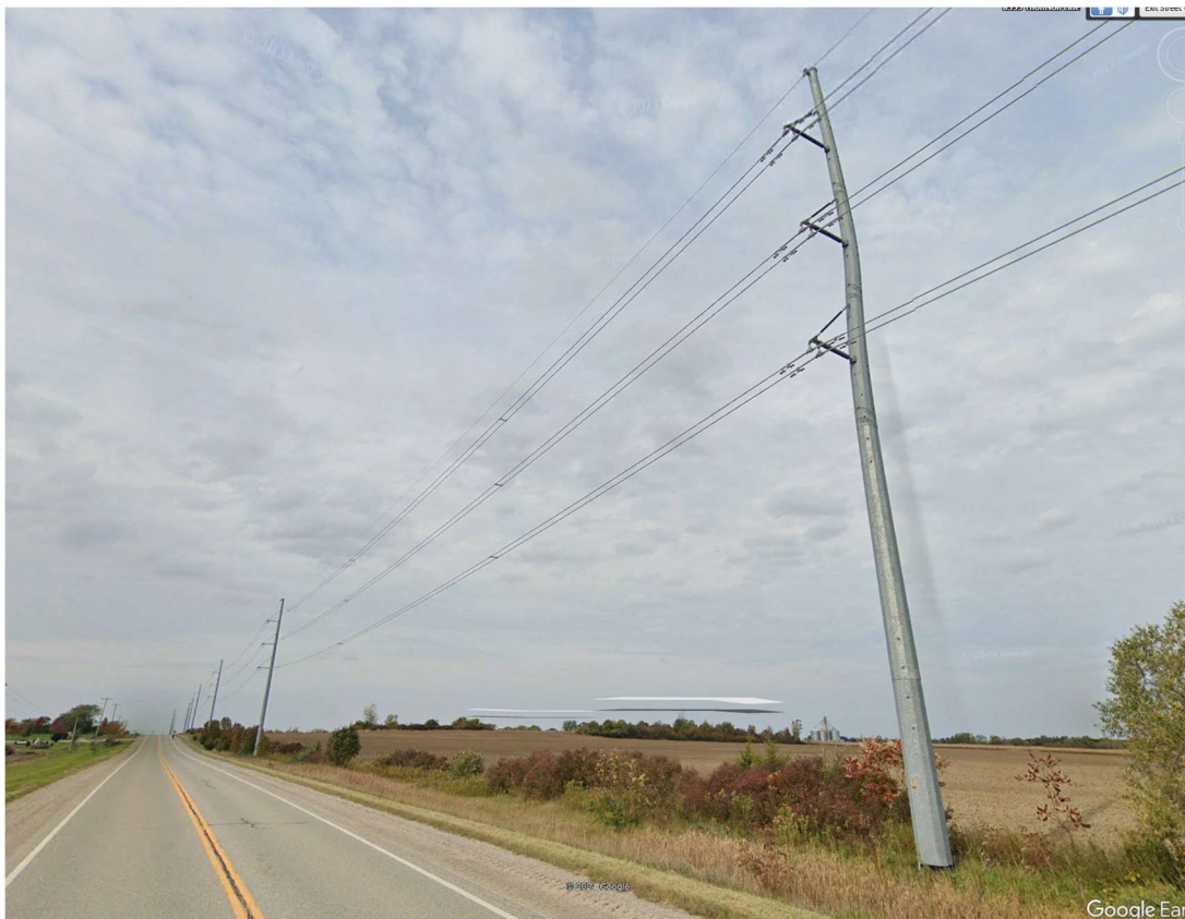
Figure 3.2.1 above is an example of a 230 kV monopole T-Line similar to the Trail Road design
