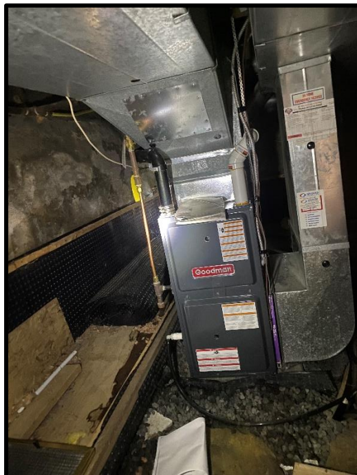
Photograph 8: View of the natural gas forced air furnace inside the 339 Roosevelt Avenue dwelling.
