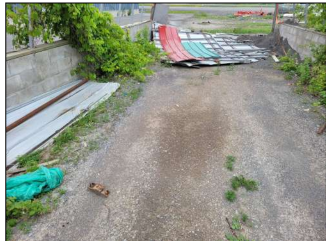
Photo 12: Stained soil in shed area.
