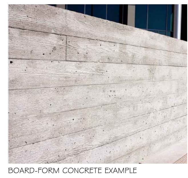
BOARD-FORM CONCRETE EXAMPLE
