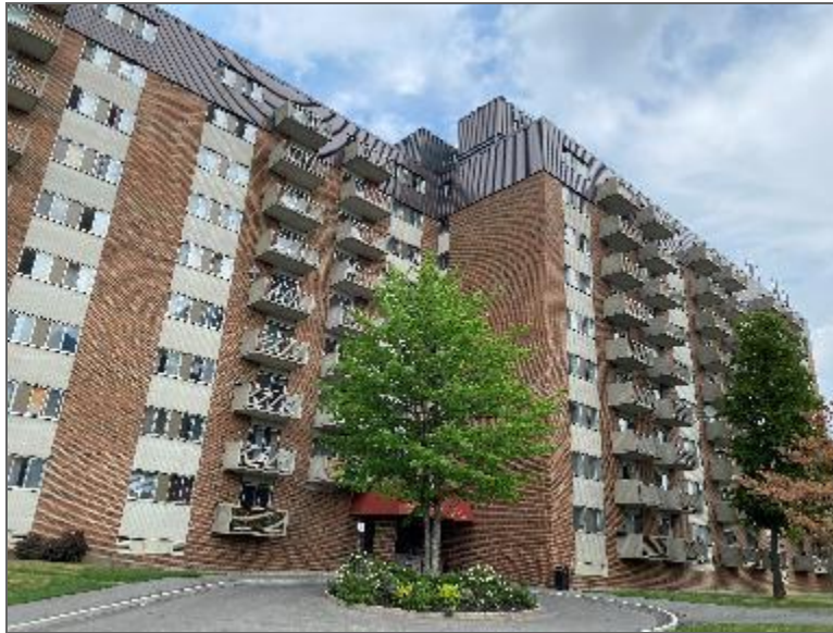
Photo 1 – Site Building A (south elevation).
