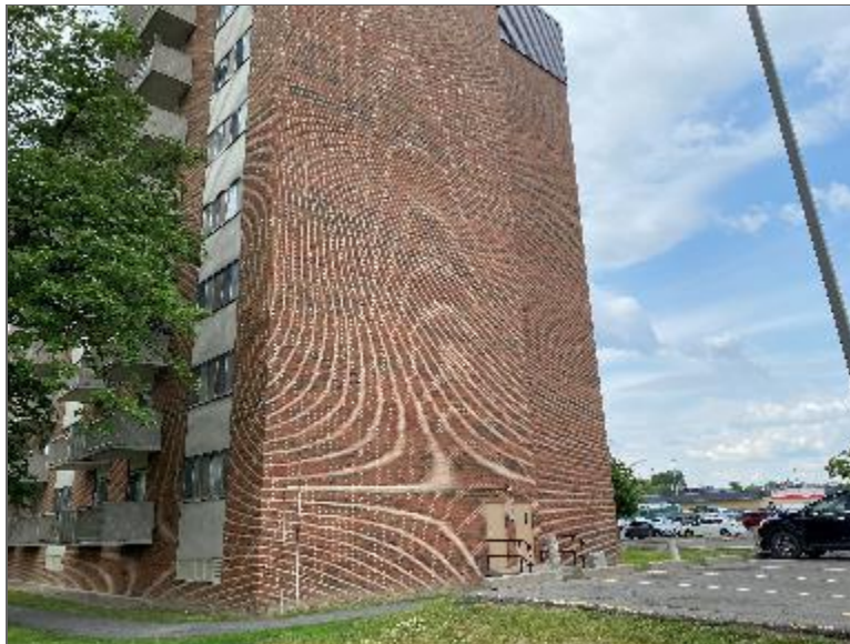
Photo 2 – Site Building A (east elevation).
