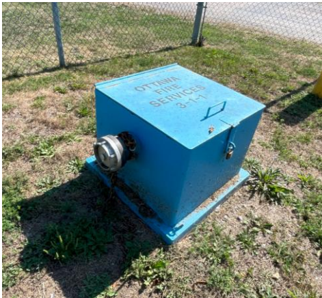
Water Supply Fire Department Connection at 8 th Line Road
