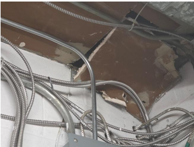
Figure 2: Service Room Ceiling and Service Penetrations Requiring Repair
