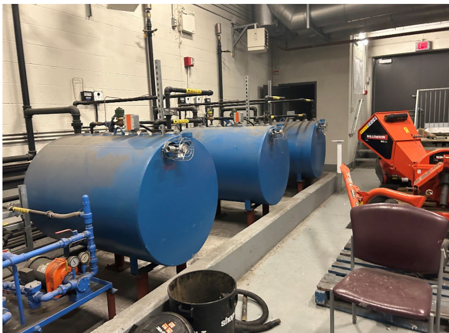
Photo 9 General view of the diesel ASTs located within the emergency generator room of Site Building B, July 8, 2025.
