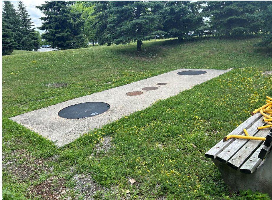
Photo 7 Diesel UST located adjacent to the east of the generator room of Site Building B, July 8, 2025.
