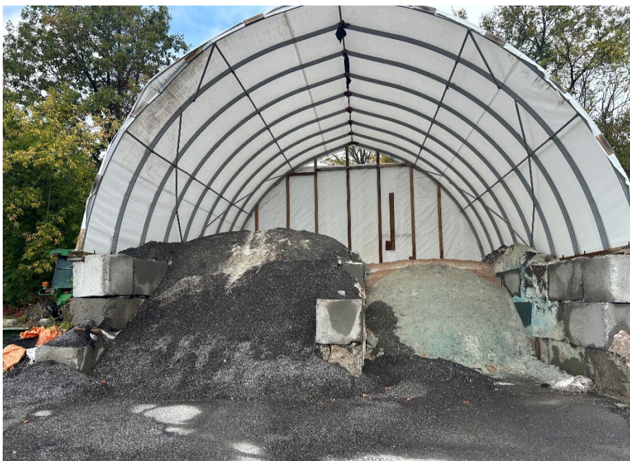
Photo 12 General view of the steel-framed, fabric-covered, road salt and sand storage structure, located on the north portion of the Site, July 8, 2025.
