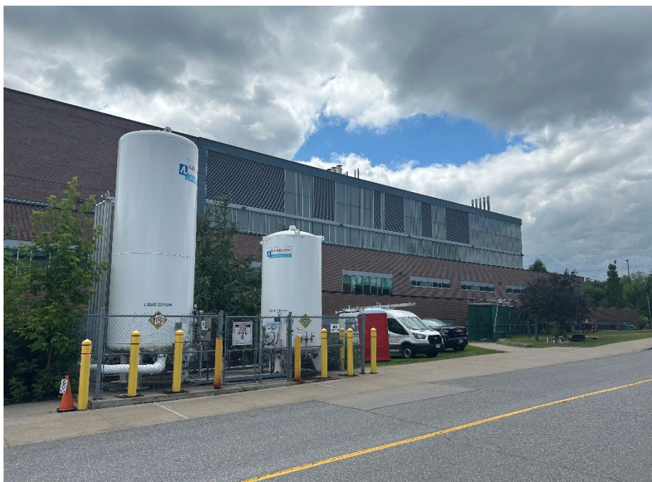
Photo 10 General view of the liquid oxygen ASTs located adjacent to the north portion of Site Building A, July 8, 2025.
