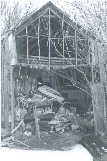
West Entry to Barn
