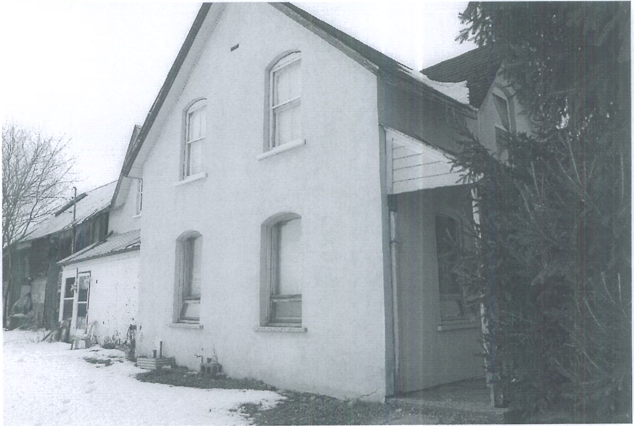
Single Family Dwelling facing South
