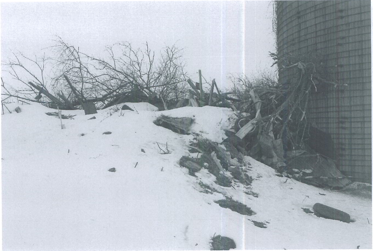
Debris Pile Adjacent Silo
