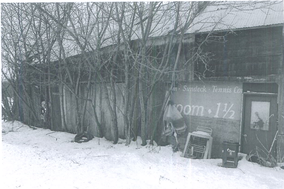
South Side of Storage Barn
